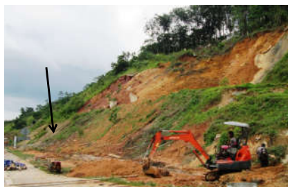
Installed Horizontal drains
