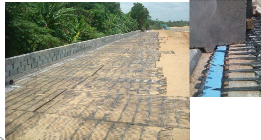
Facing blocks and Geogrid Reinforcements Placed
