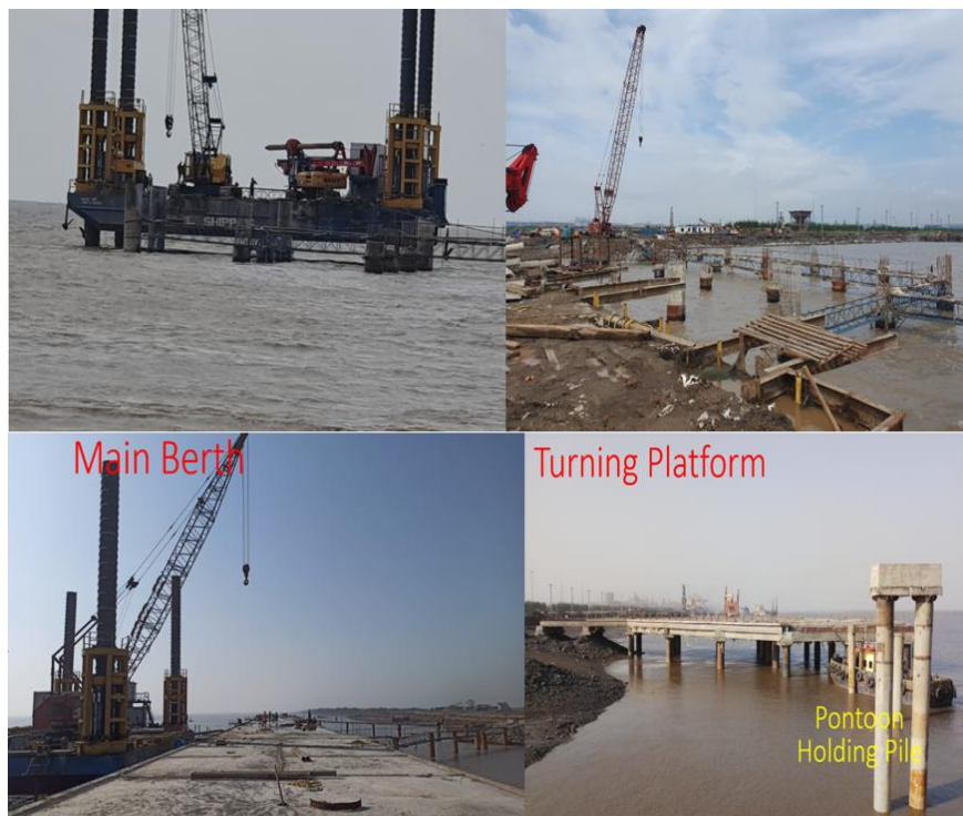
Fig.33. Stages of construction of RO-RO Facility at Hazira
