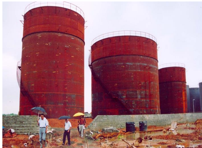
Fig.7. Completed tank farm
