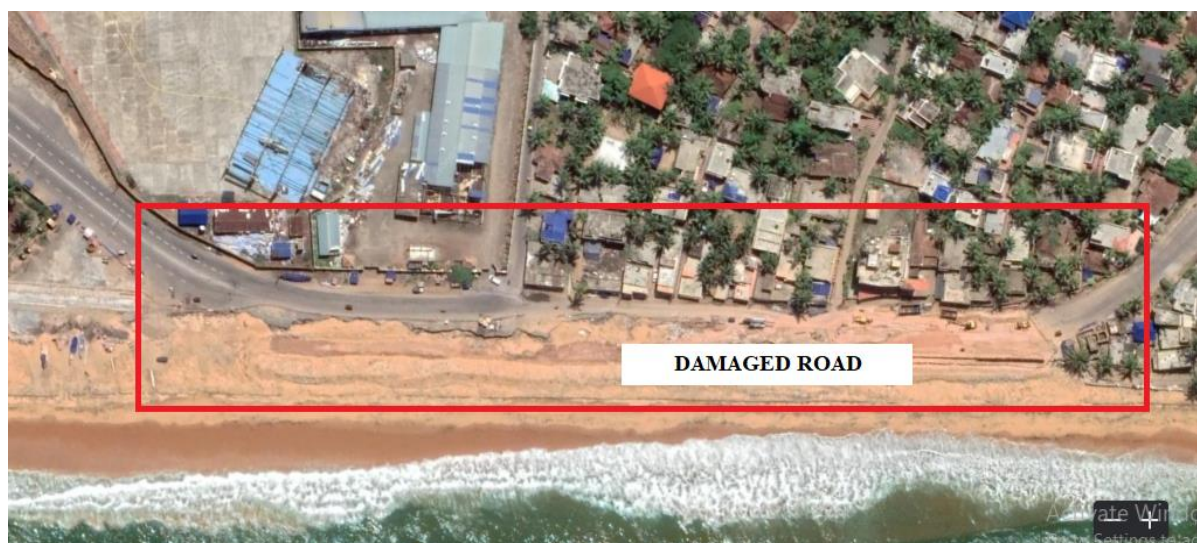
Fig.12. Damaged road of Shanghumugham beach
