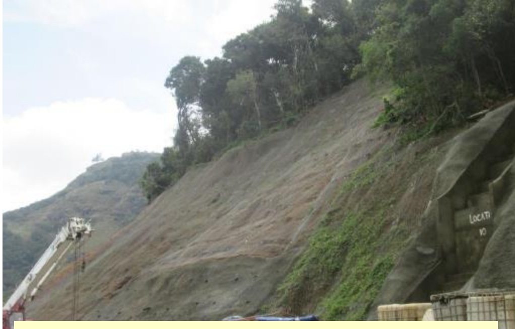
Nail heads connected with high tensile wire mesh and coir mesh for hydroseeding
