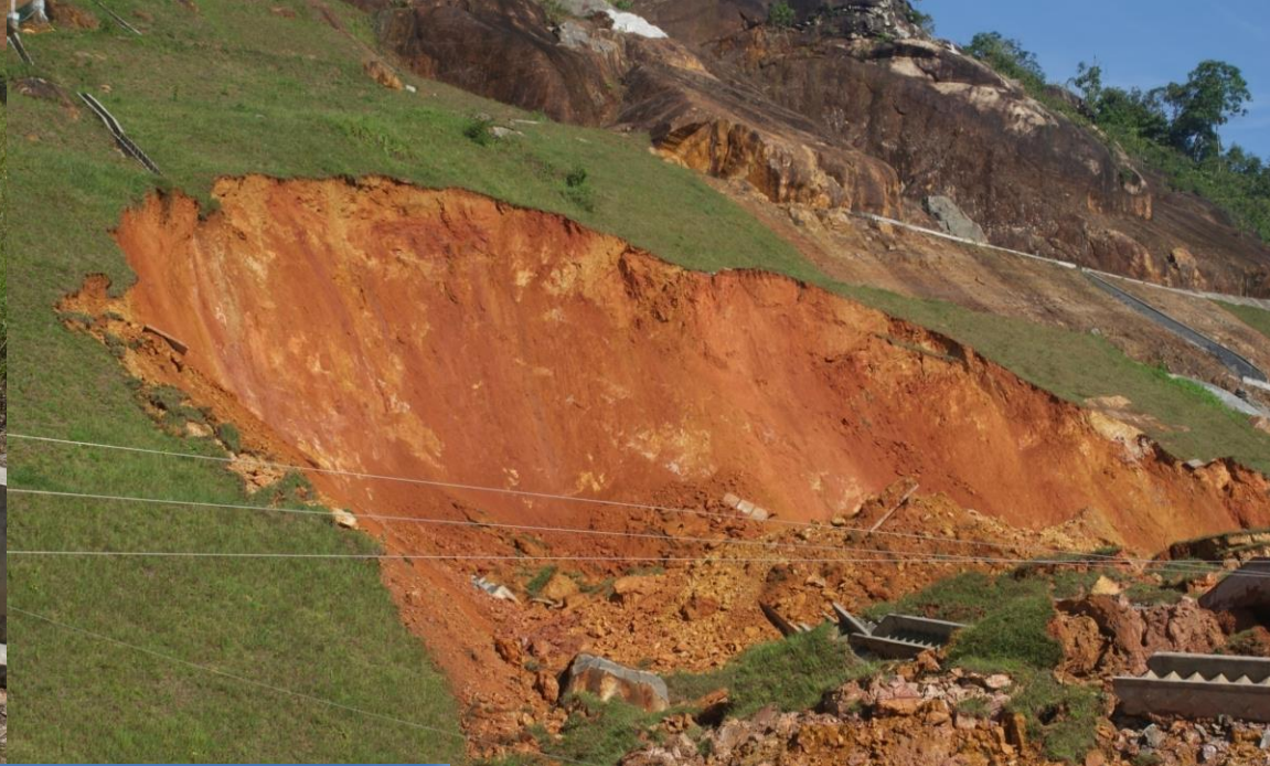
Whitish clays of low shear strength appearing in the failure surface
