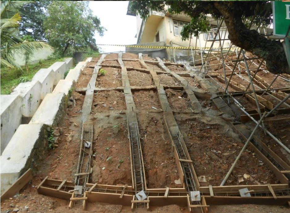
Soil Nailing with beams connecting nail heads and vegetation Mahamaya College - Kandy
