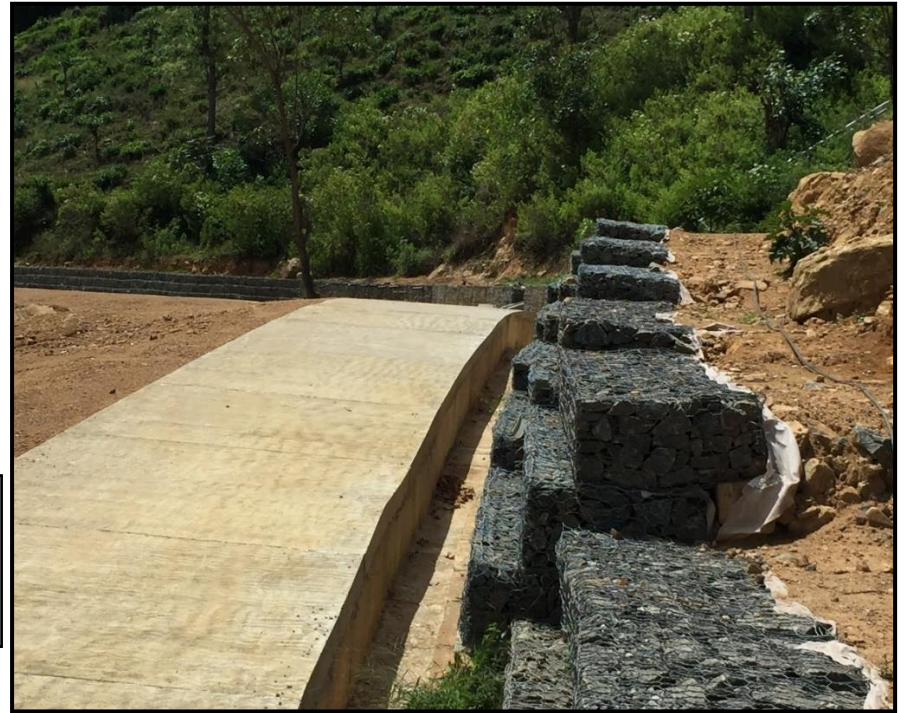
Earth removal and slope protection
