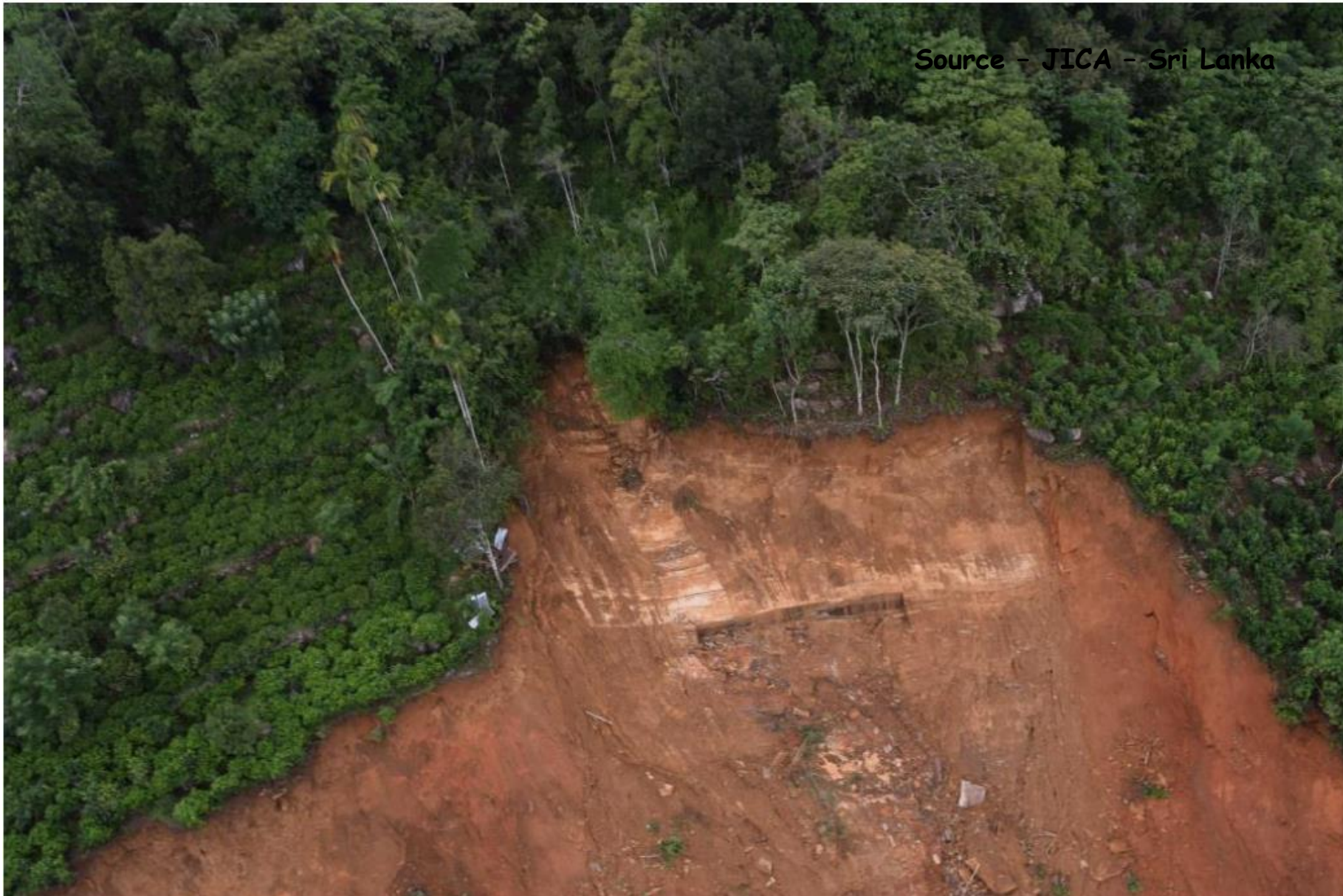
The crown of the landslide - An aerial view
