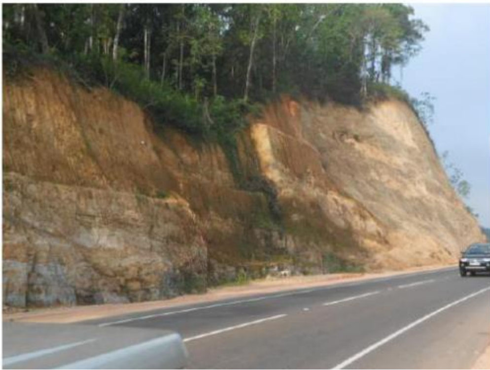
Immediately after cutting 24-3-2014
