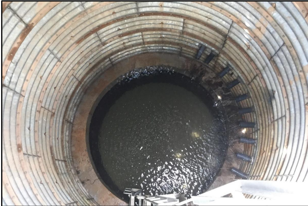
Figure 4.13 : Inside a drainage well (B2, C2, C3, D3, D4 in figure 4.9)
