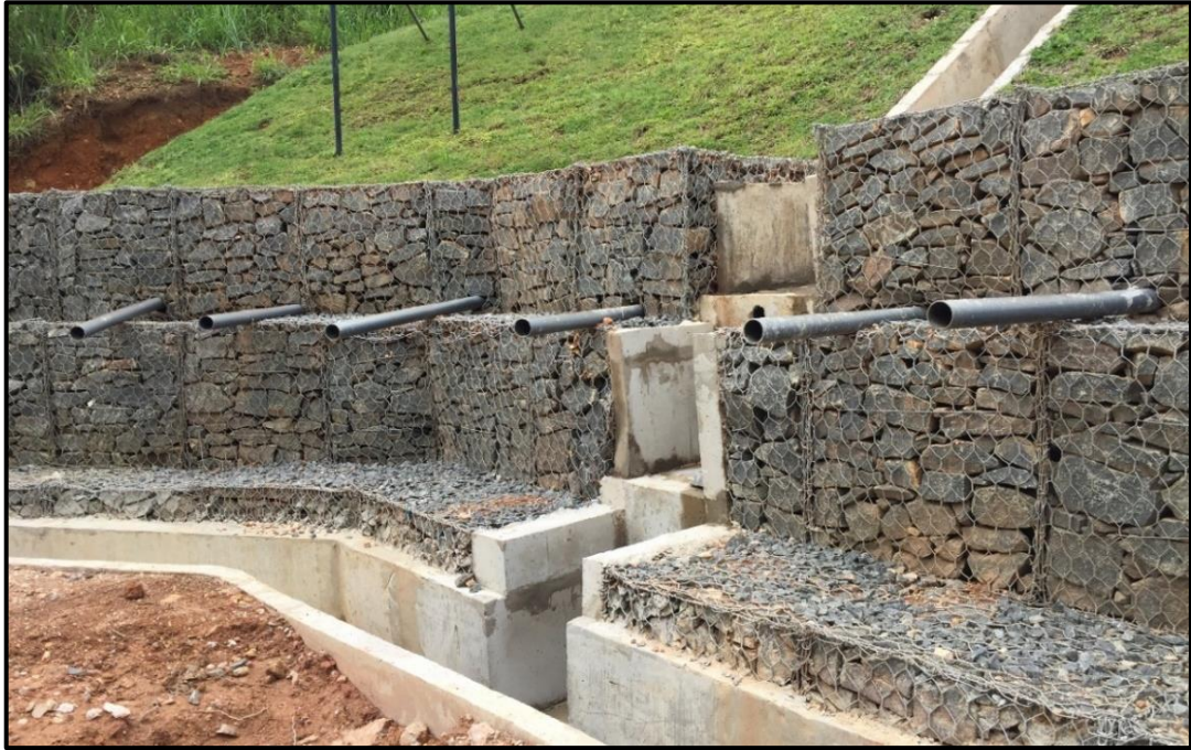
Figure 4.12: Horizontal drain outlets at toe area (B1, B2 in figure 4.9)
