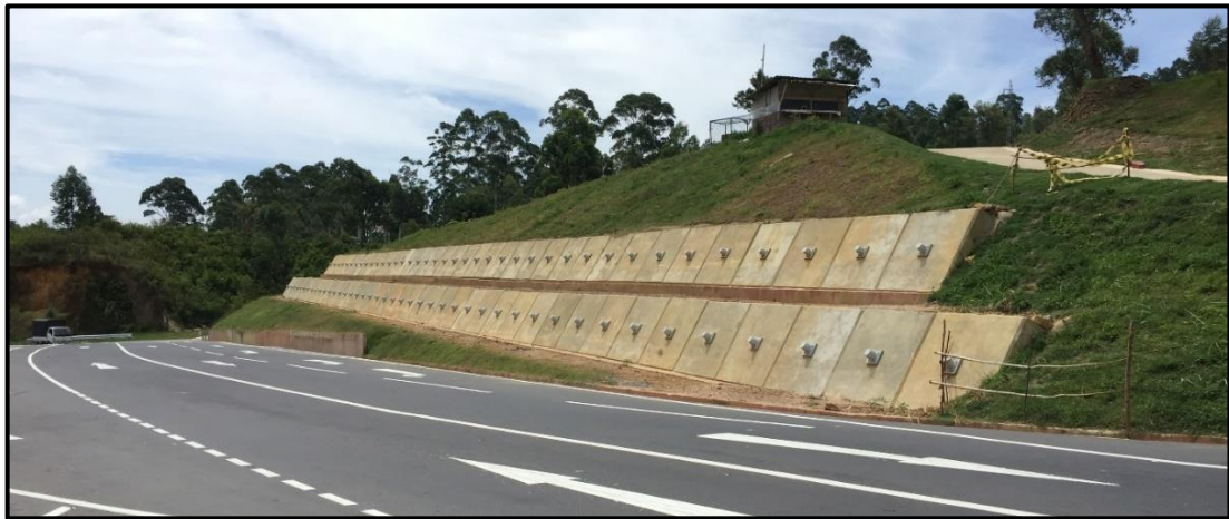
Figure 4.15 : Ground anchor beside the road (C2, B2, B3 in figure 4.8)
