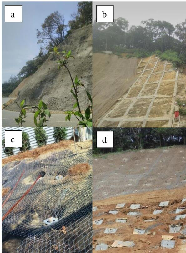
Fig. 1 (a) Full-face shotcrete, (b) Concrete grid beams, (c) High tensile steel wire mesh with metal bearing plates, (d) High tensile steel wire mesh with isolated reinforced concrete nail heads
