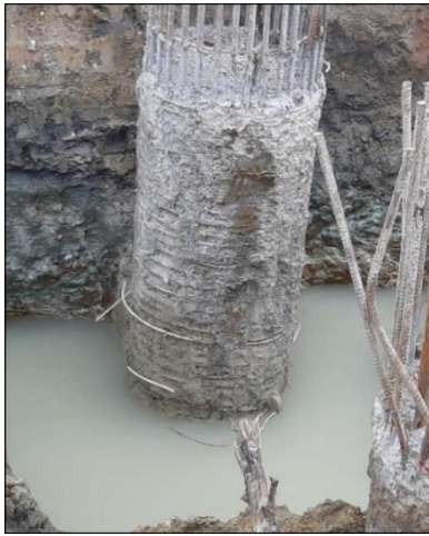
Fig. 2 Surrounding excavation of pile A
