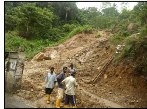
Fig. 2 Failure just after the rainfall event
