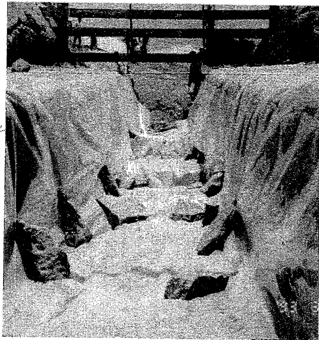
Fig 10 : Sealing of boundary shear surface and construction of trench drain using geosynthetics as an interim control measures.
