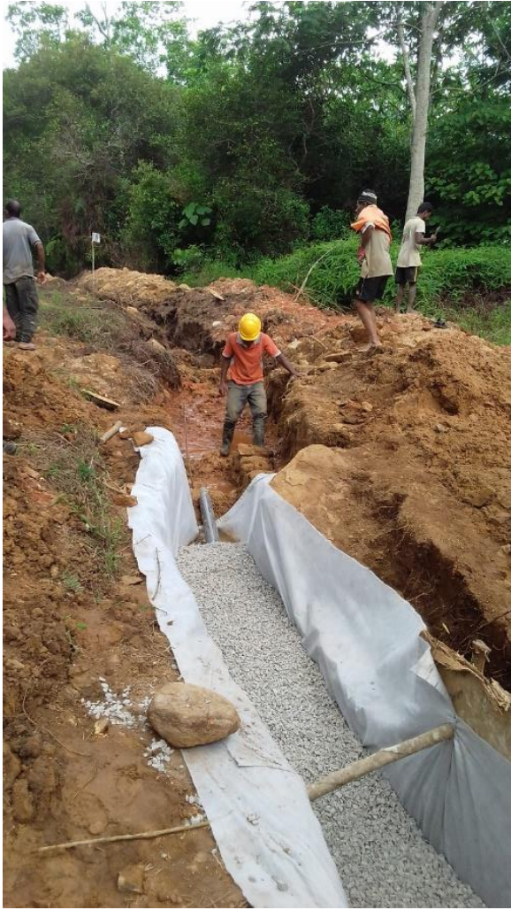
Construction of Trench Drains
