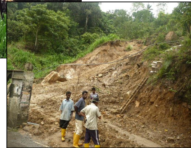
Just after the Failure
