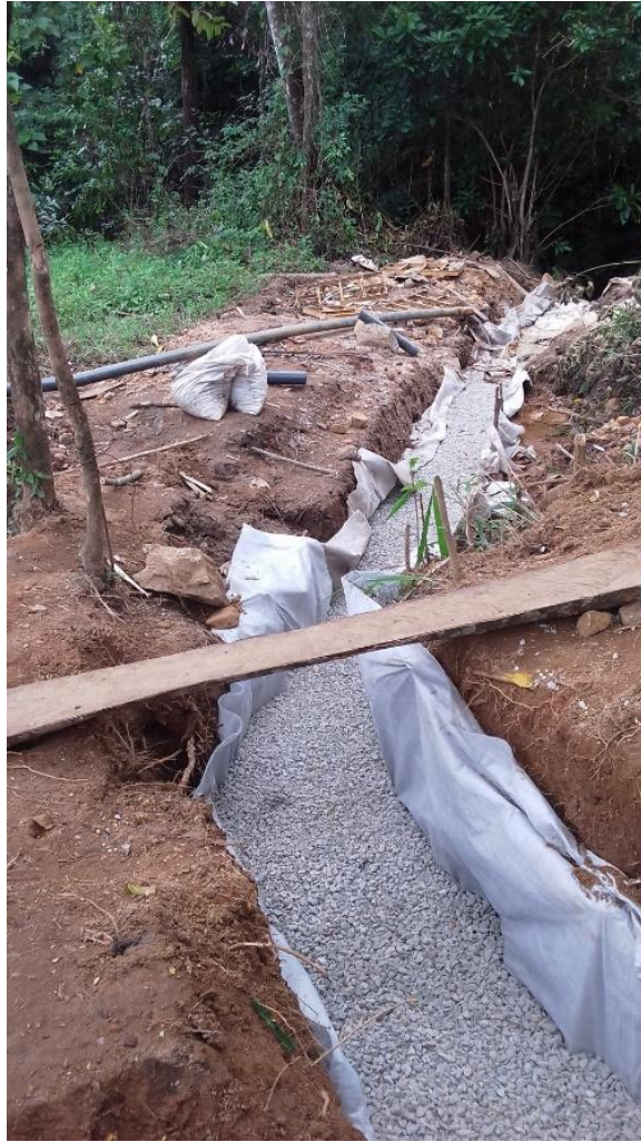
Construction of Trench Drains
