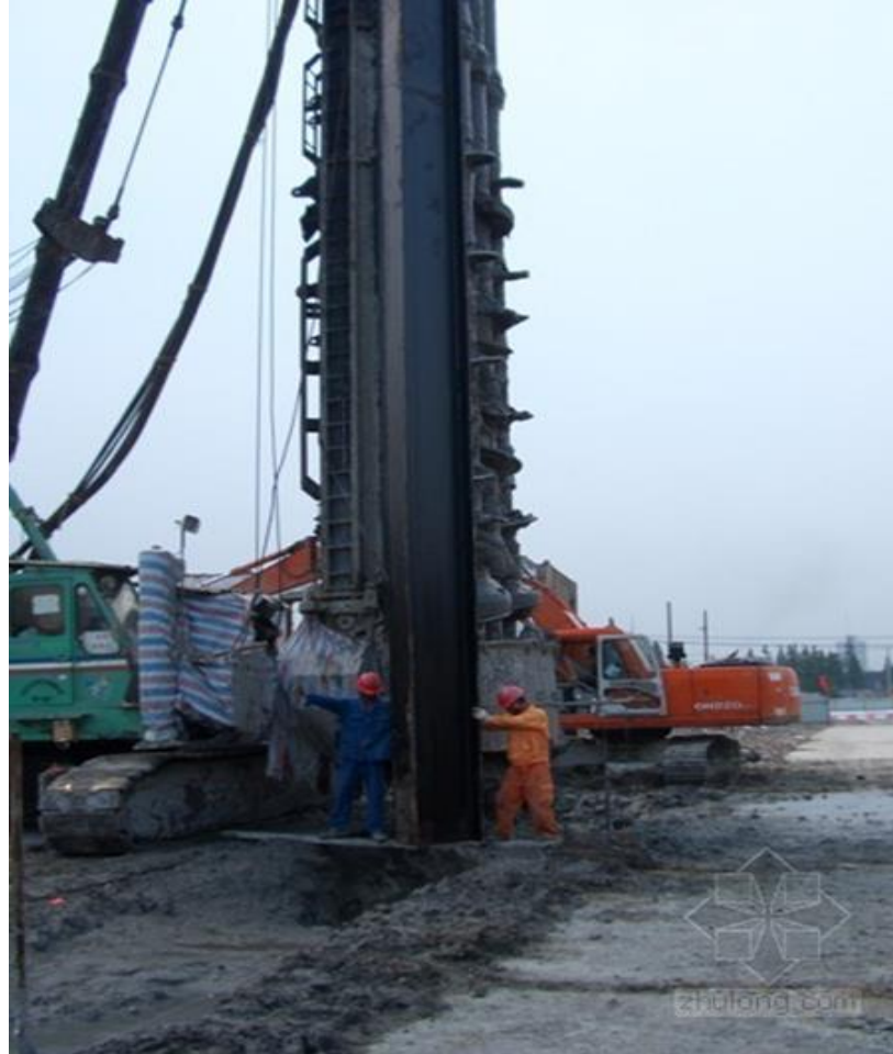
Inserting H-Beam
