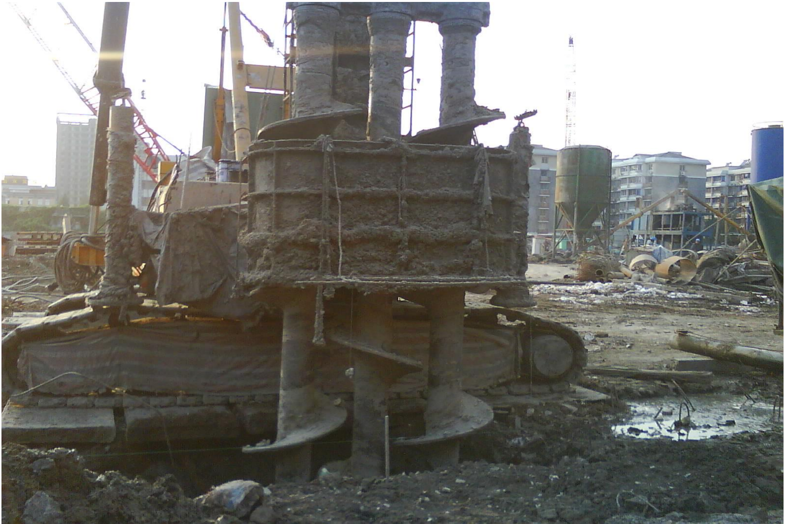
Soil mixing machine
