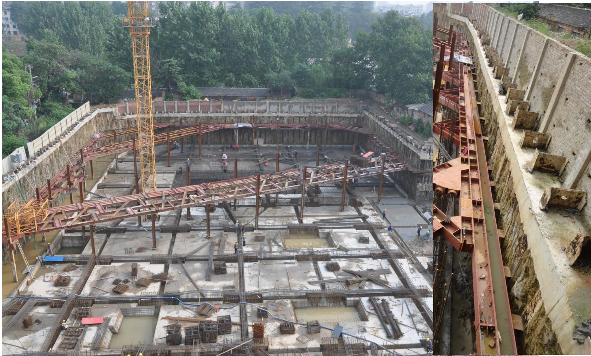
Nanjing Central Jindi excavation (SMW + steel frame strut)
