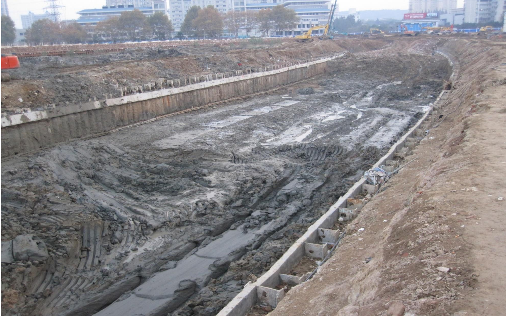
Wuhan Donghu tunnel (SMW + anchor)
