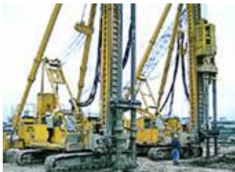
Ground Solidation Rig
