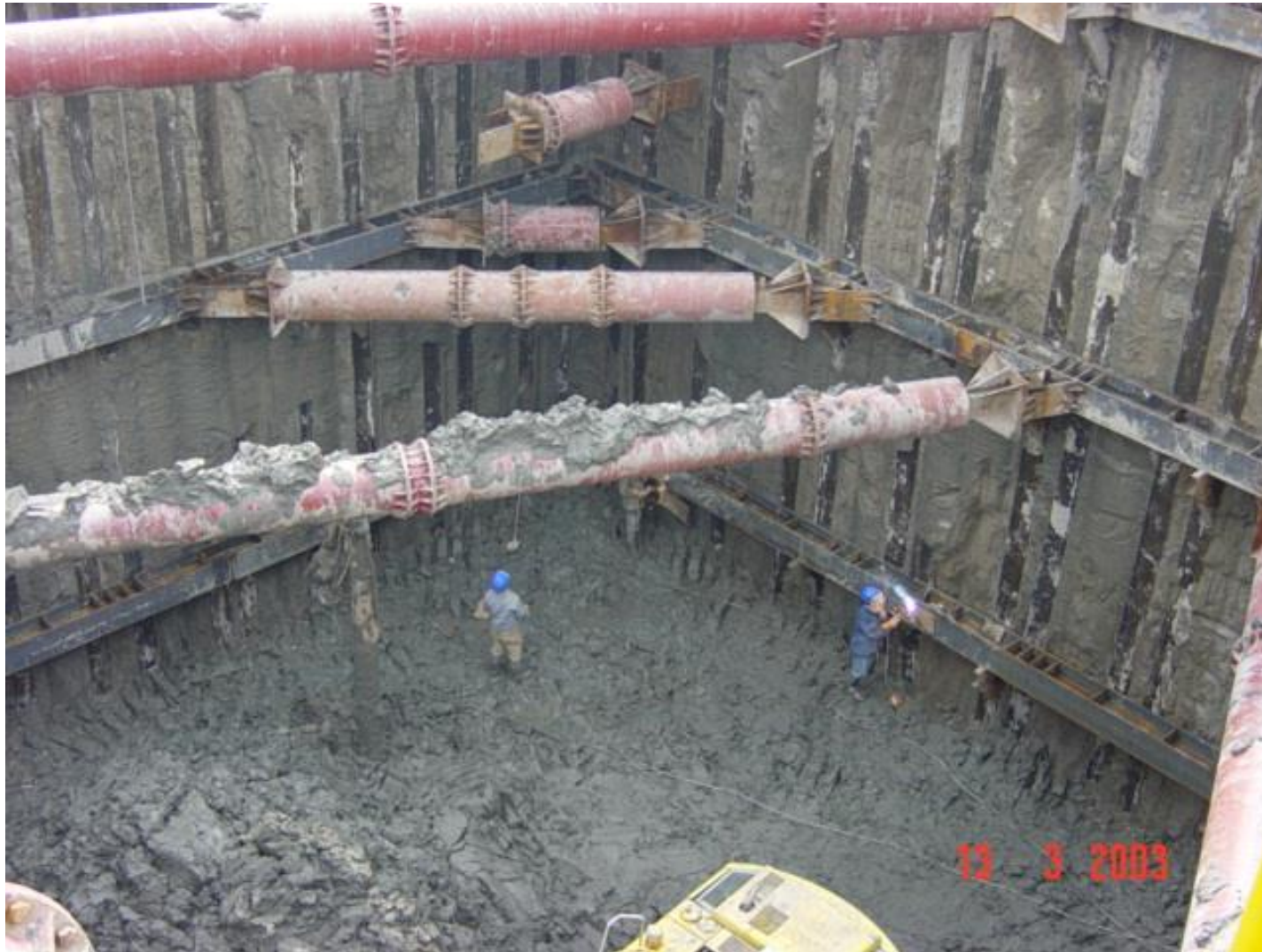
Shanghai South railway station excavation (SMW + steel pipe strut)
