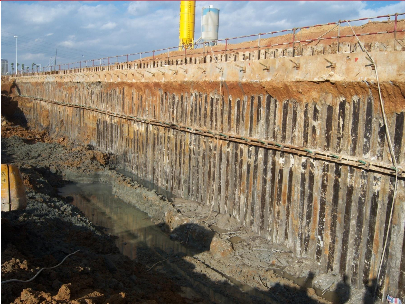
Kunming tunnel ((SMW + anchor)
