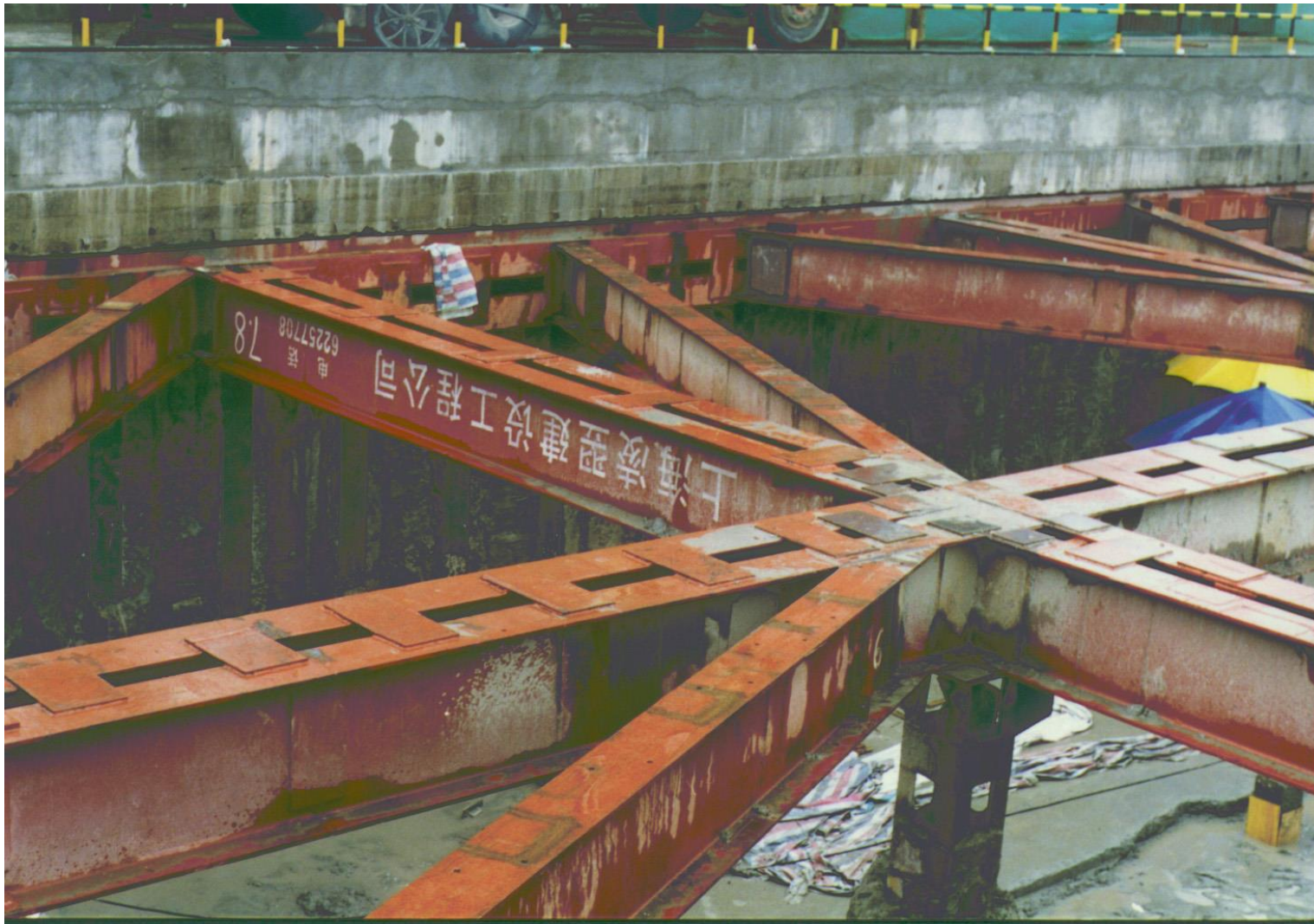
Shanghai Delong Plaza excavation (SMW + steel beam strut)
