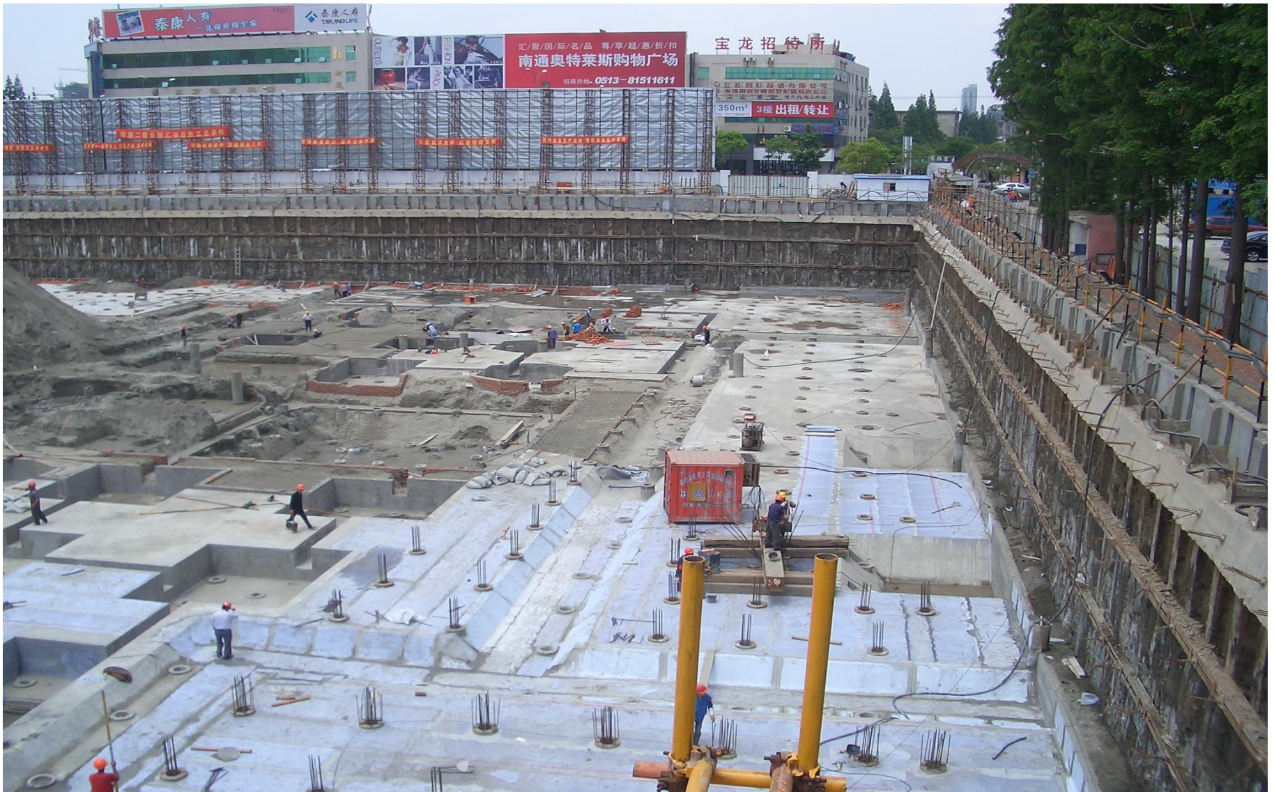
Nantong cross street excavation ((SMW + anchor)
