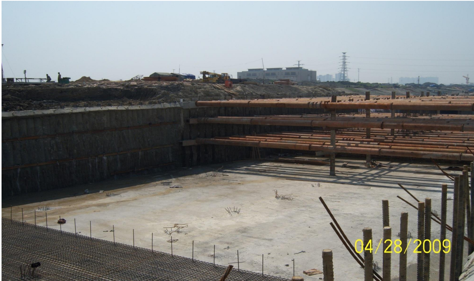
Wuhan Wenling tunnel (SMW + steel pipe strut)
