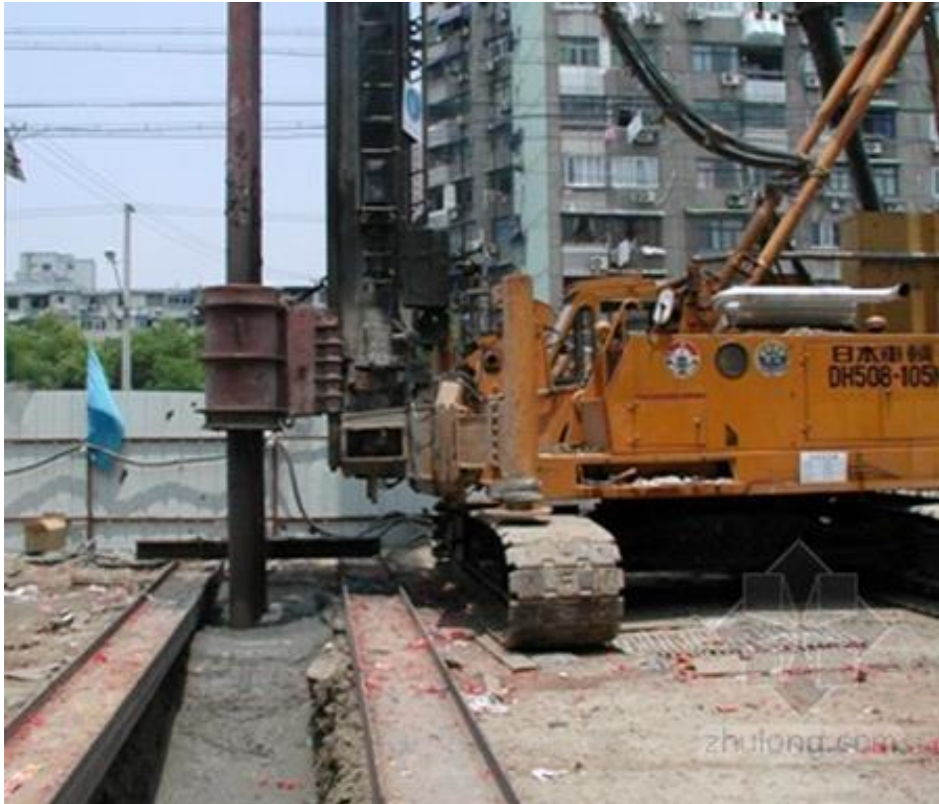
Soil mixing machine
