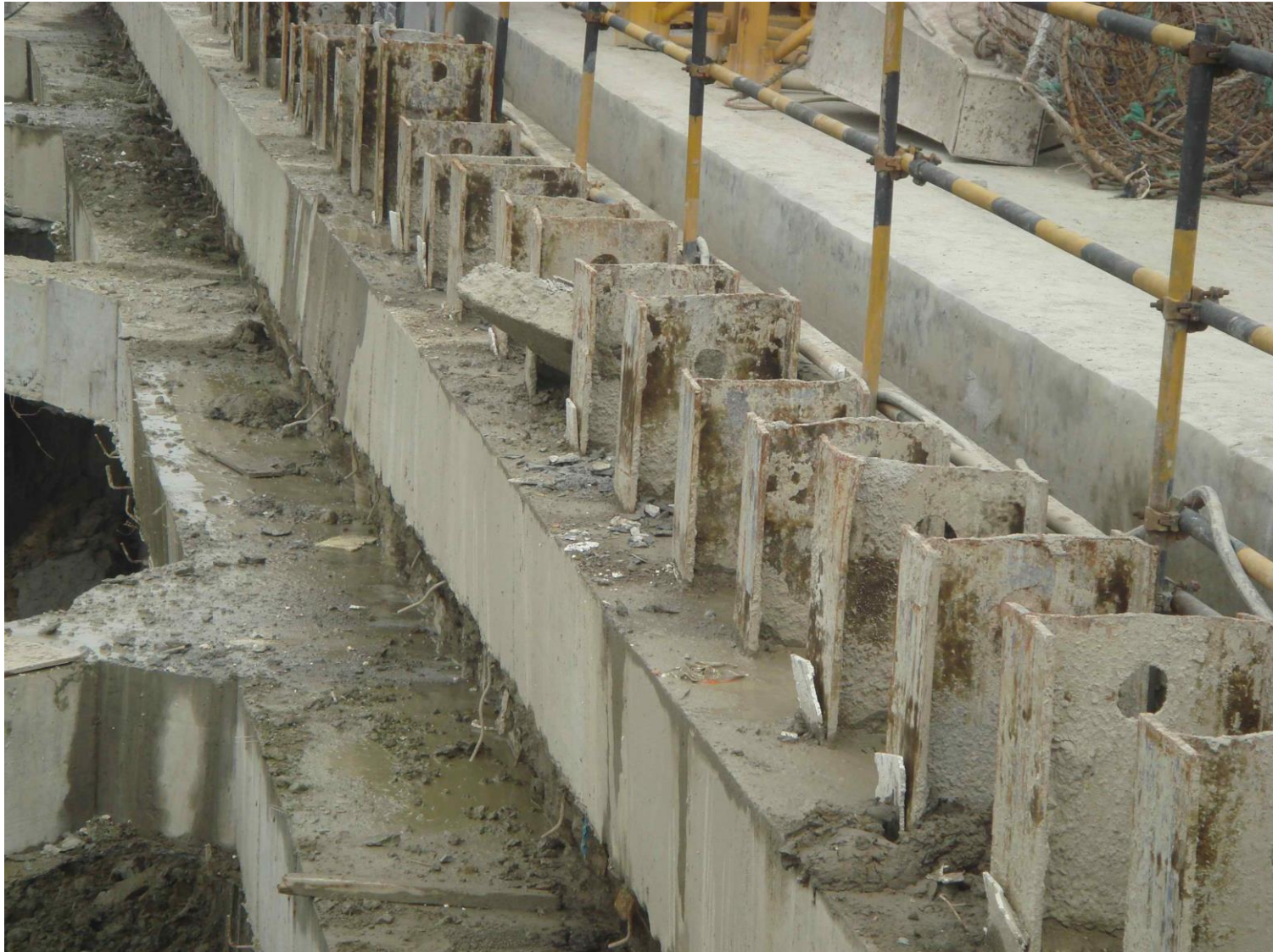
Finished SMW retaining wall
