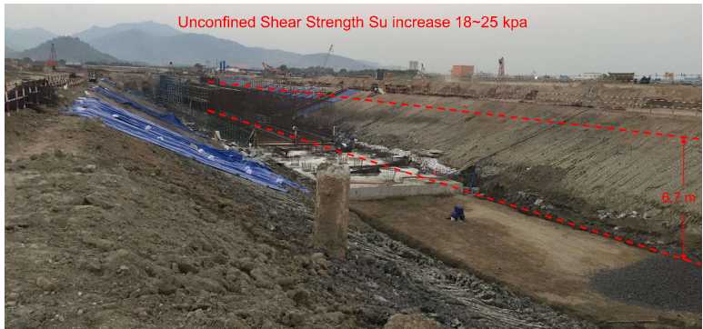
Excavation up to 6.7 m without retaining wall
