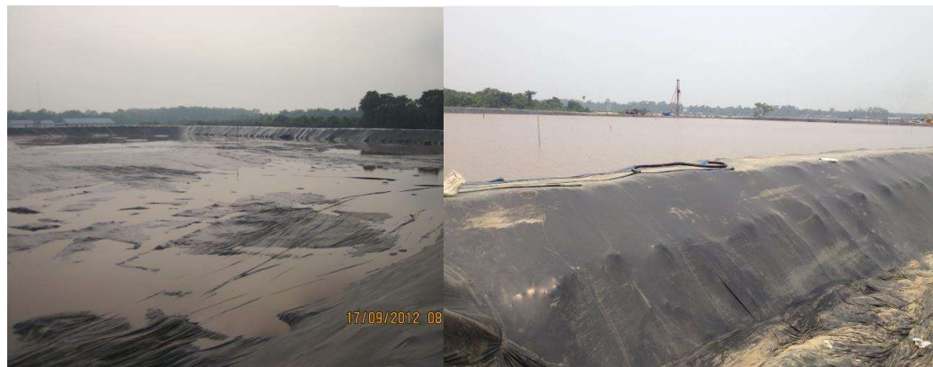
Water Surcharge Fill During VCM
