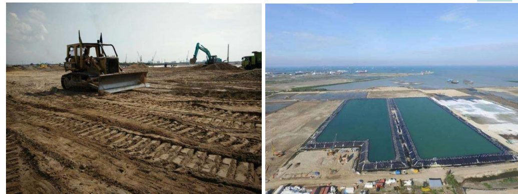
Soil + Water Surcharge Fill During VCM
