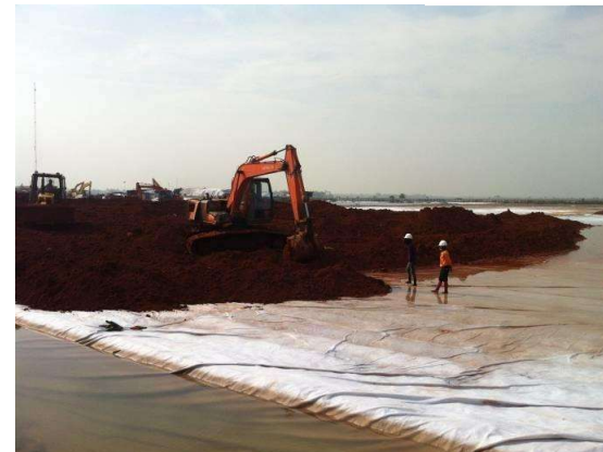
Soil Surcharge Fill During VCM
