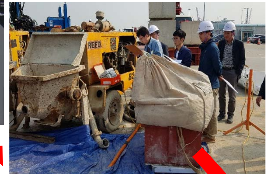
3. Measure discharged quantity on scale
