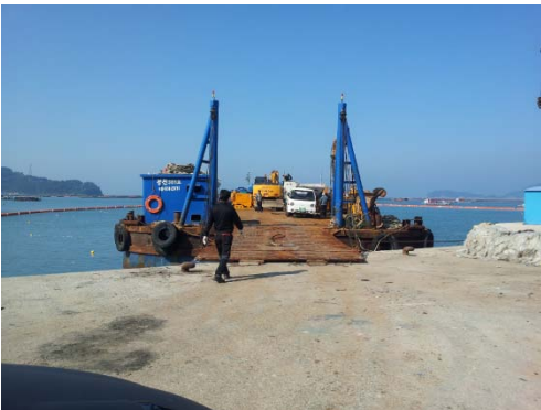
Injection equipment setting on barge
