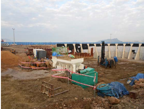
Injection equipment setting on land
