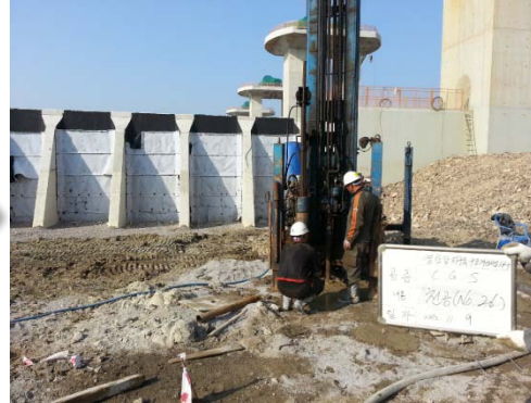
Drilling on land
