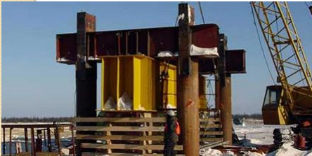
Anchor pile system
