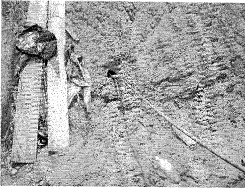
Grouting nearing completion
