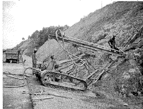
Drilling the hole for the installation of the Nail
