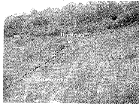
Landslide at Bogahagoda (Souther part of STDP 36+) State of the Cut Slope prior to Failure
