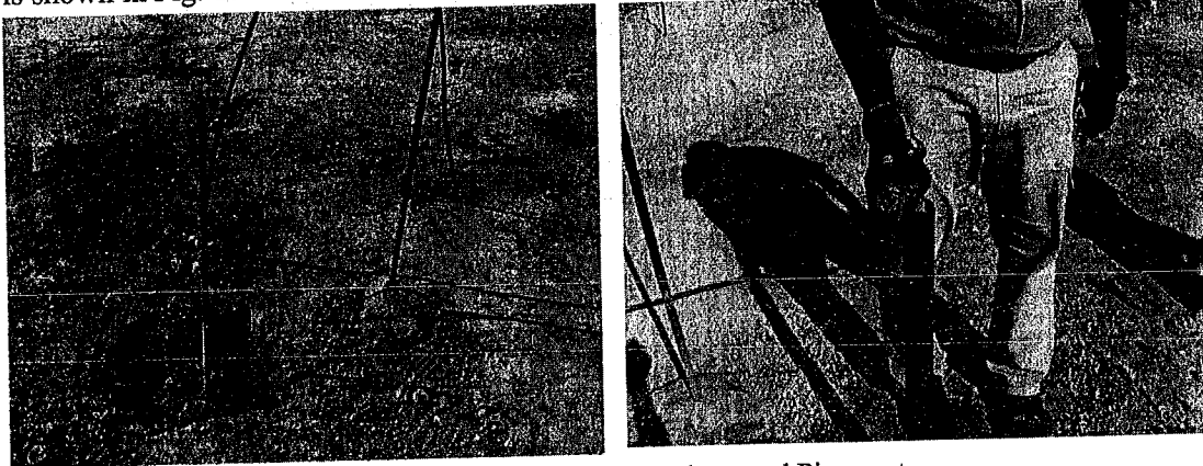
a Installation of Settlement plates and Piezometers
