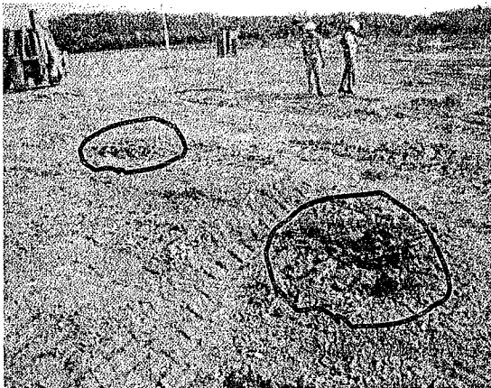
a. Some spots where soft soils had oozed out from the platform
