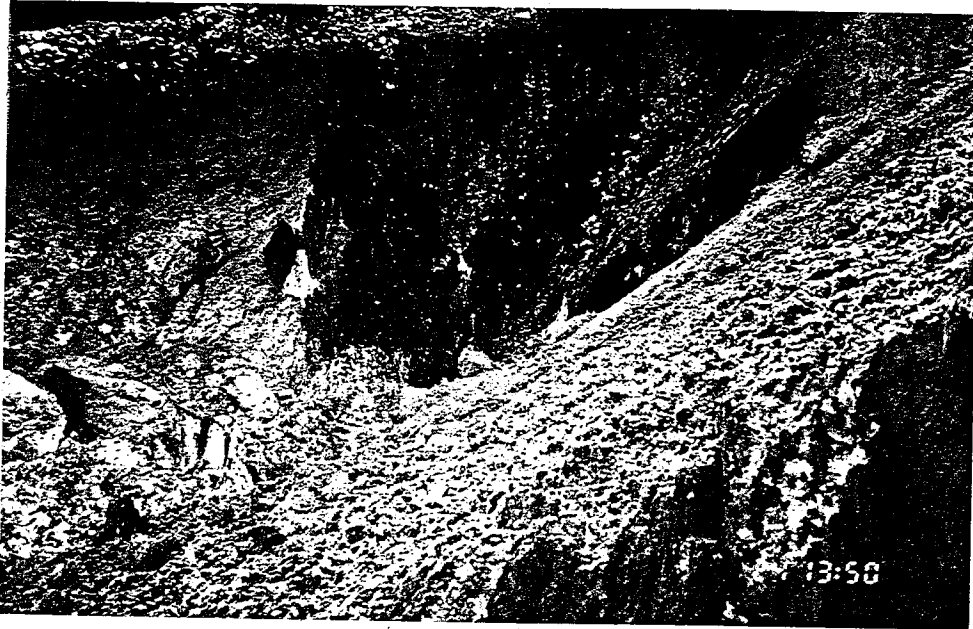
Fig. 4 Earth failure on residual formation.
