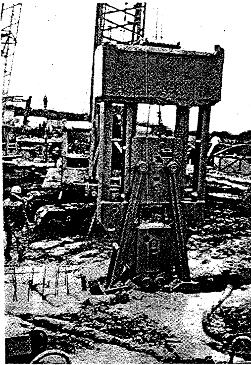
Clam Shell Excavation Slurry trench panel
