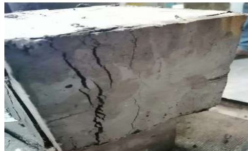
Figure 10 (b) Crack pattern of cubes
