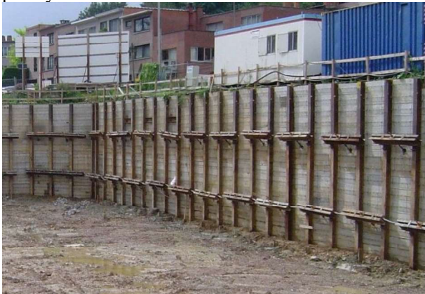
Fig 8: Actual excavation with soldier pile wall
