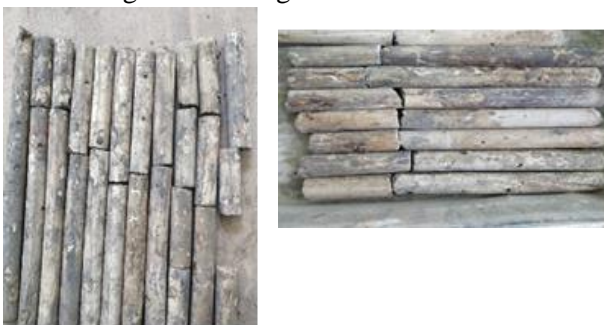
Fig. 5. Failed Soil Cement Columns
