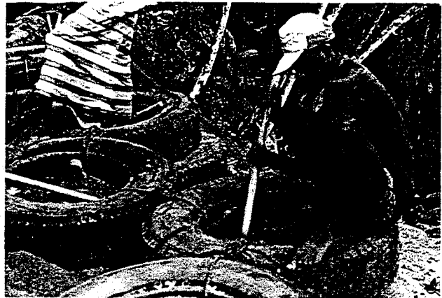
Plate 2 - Compaction of Fill Inside the Tube Space
