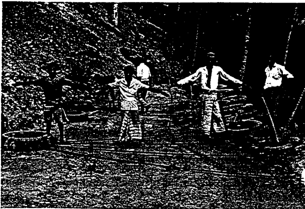
Plate 1 - Placement of Anchor and Facing tyres
