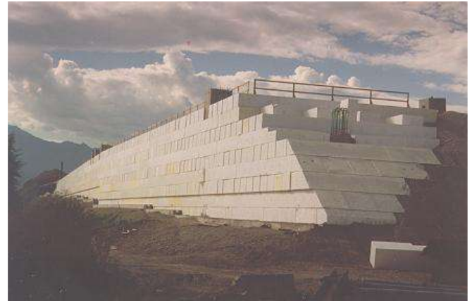
Figure 5. Geofoam embankments at the Port of Brisbane Motorway in Brisbane
