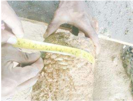
Figure 11: on site measurement of grouted body of pulled out test nail
