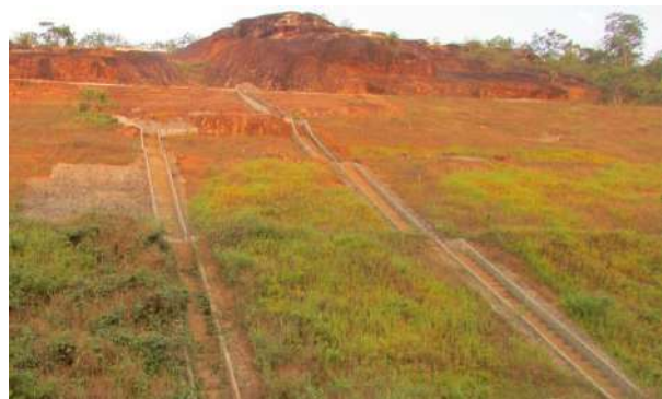
Figure 4: Berm drains and cascade drains
