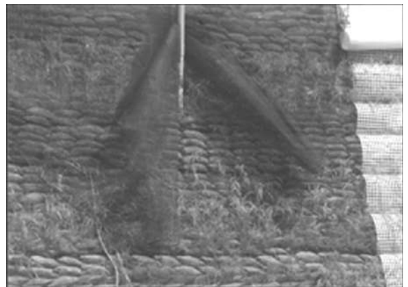
Figure 9. The wrap face construction of geogrid reinforcement
